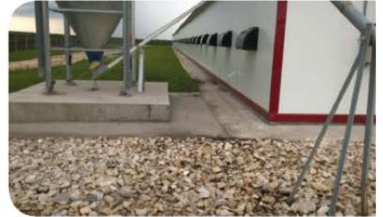
Exterior free of debris
