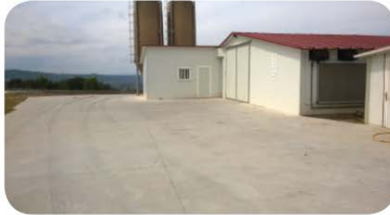
Concrete area in front of entrances
