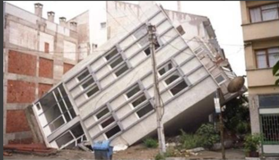
Adapazari, Turkey (August 18, 1999) Liquefaction Damage
