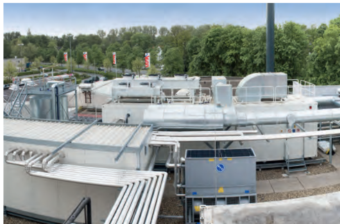
CHP for industrial bakery "Mestemacher" in Gütersloh / Germany: GR 849 N5 // Electr. power: 849 kW // Therm. power: 948 kW // Cooling cap.: 105 kW
