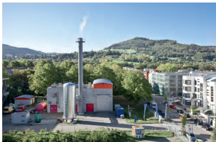
CHP for housing estate "Vauban" in Freiburg / Germany: GR 849 N5 // Electrical power: 849 kW // Thermal power: 1,300 kW
